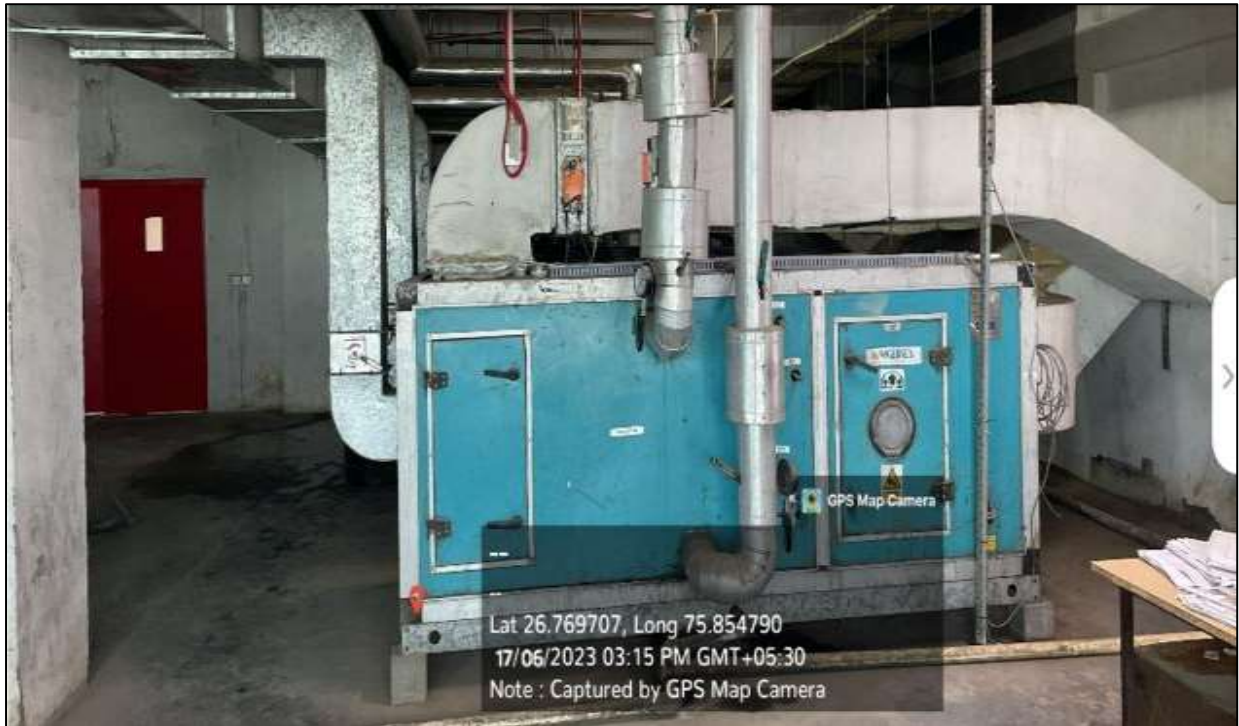
Figure 15 AHU (Air Handling Unit)
